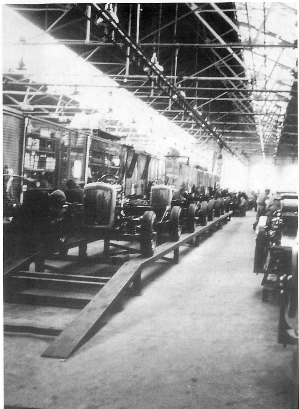
Early TA 21 chassis on the production line at the Works in 1950.
