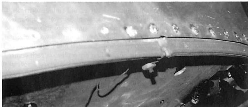
Attaching panels by welding through 8mm holes
